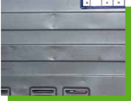
Abrasions, scuffing and scratches on the loading floor caused by transportation of goods or loading activities.
