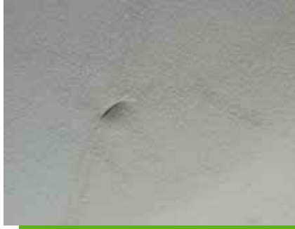
The headlining of the driver's cabin shows minor damage, but is not influenced in its function.
