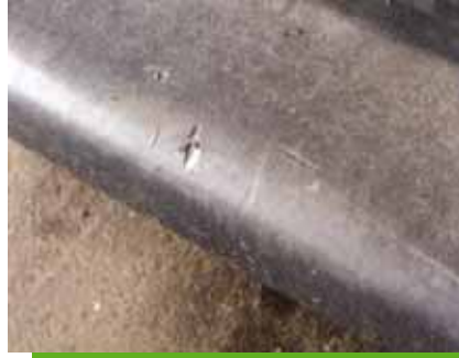
Damages to the sills of the loading compartment caused by loading of goods and not infringing on the function of bumpers, lights, number plates, etc.
